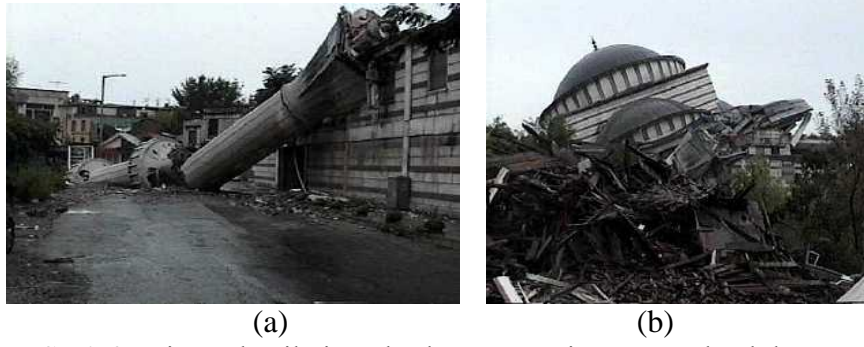
Şekil 2. Minare devrilmiş ve kırılmış ve cami yan yatarak yıkılmış. Figure 2. The minaret is overturned and broken and the mosque is lying down on its side
